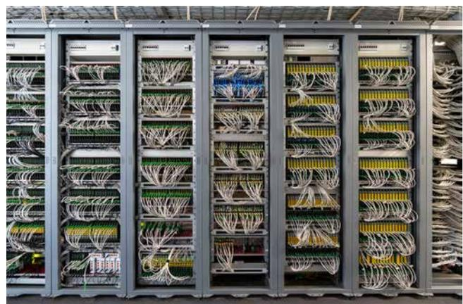
**FIGURE 6** – Rack cabinets with several types of ONU used in load tests
